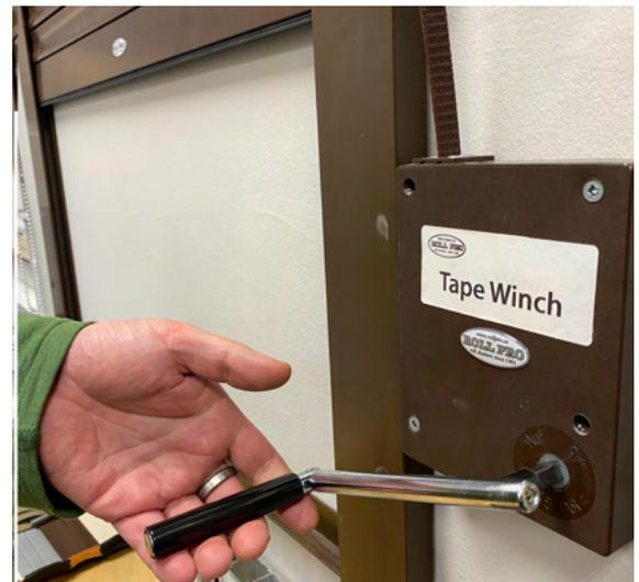
**Tape Coiler** (or tape winch for shutter with large width)
